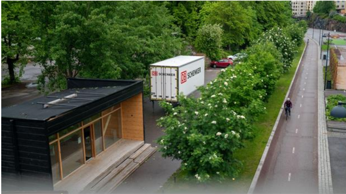
FIGURE 9 CONCEPT OF MICROHUBS HAS BEEN TESTED IN HELSINKI IN EARLIER PROJECTS (SMUD AND LMAD)
